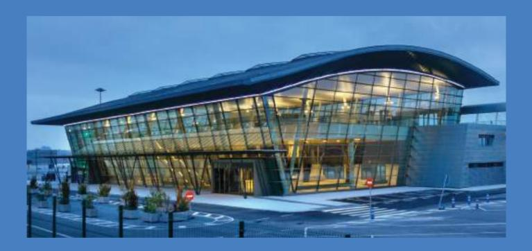
Measuring 15 metres in height and with 3,200 m<sup>2</sup> of floor space, it was conceived as a huge, crystalline container with a rectangular floor plan and a sloping zinc roof, making the building light, dynamic and luminous.
